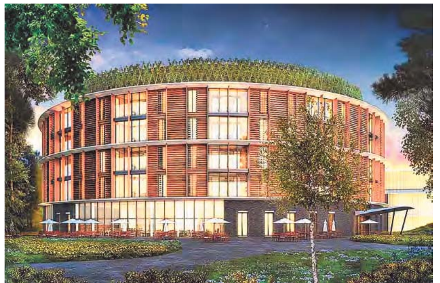
Das Bettenhaus soll 2019 fertig sein. • The ward building is to be completed in 2019.
